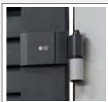
Clamp installation on window frame
