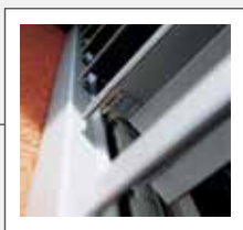
Each slat fastened individually on the side
